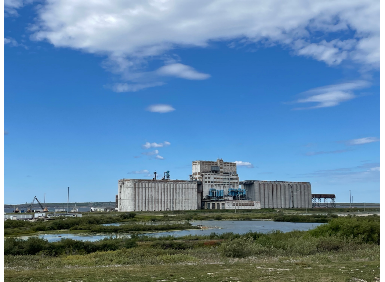
The Churchill sea port and grain elevators
