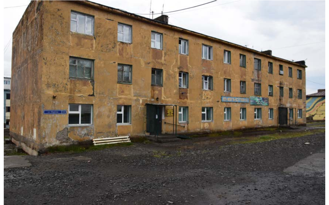
Semi-abandoned apartment building
